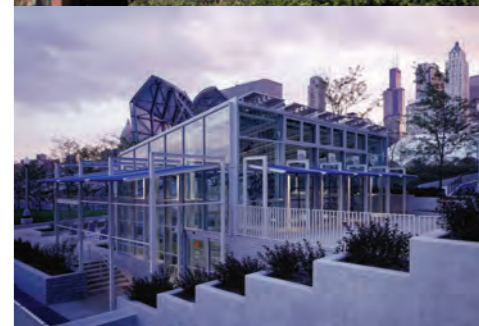
Millennium Park Bike Shelter Chicago, IL
